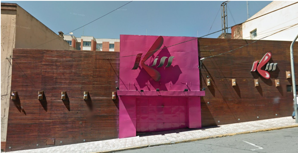
Figure6 - Facade of the Kiss Nightclub illustrating the spatial proximity of the two adjacent entrance/exit doors.
